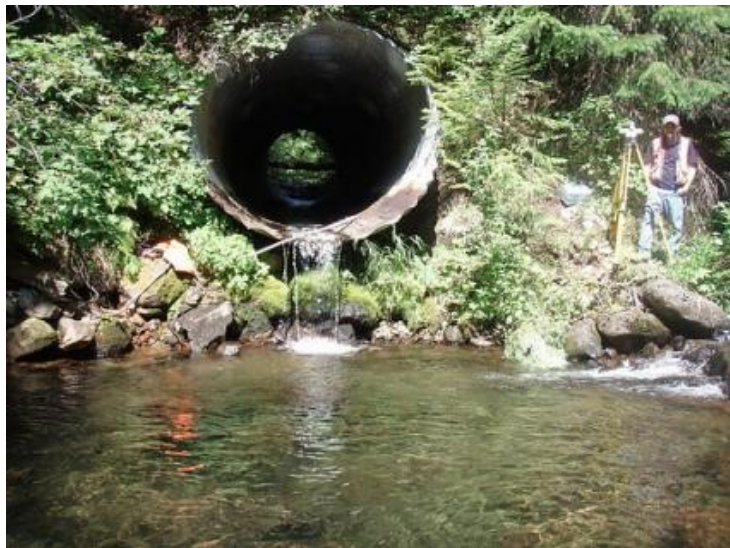
A circular culvert on the Klamath National Forest prior to being upgraded. (Photo by U.S. Forest Service.)
