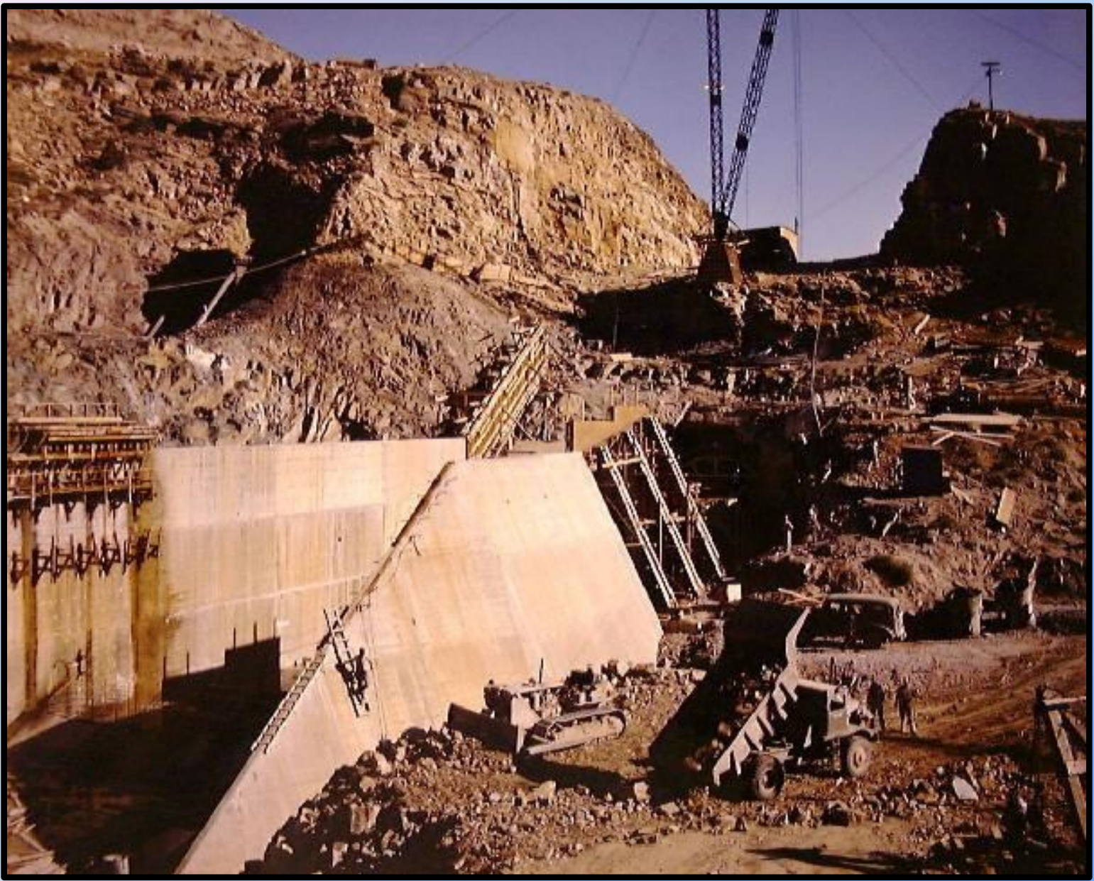
Construction of Boysen Dam on Wyoming's Wind River during July, 1949. Image made from Kodachrome 8 x 10 inch transparency. This is one of the earliest color photographs taken by a Bureau of Reclamation photographer in the State of Wyoming.
