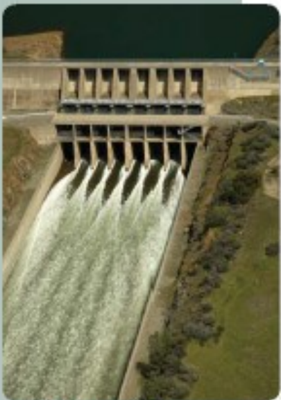
Oroville Dam Spillway high water release
