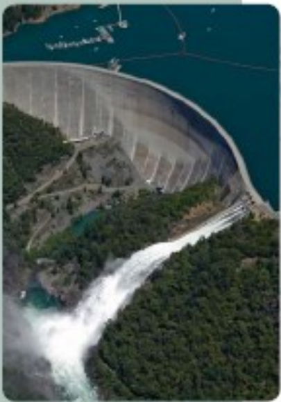
New Bullards Bar Dam Spillway releasing water into the Yuba River
