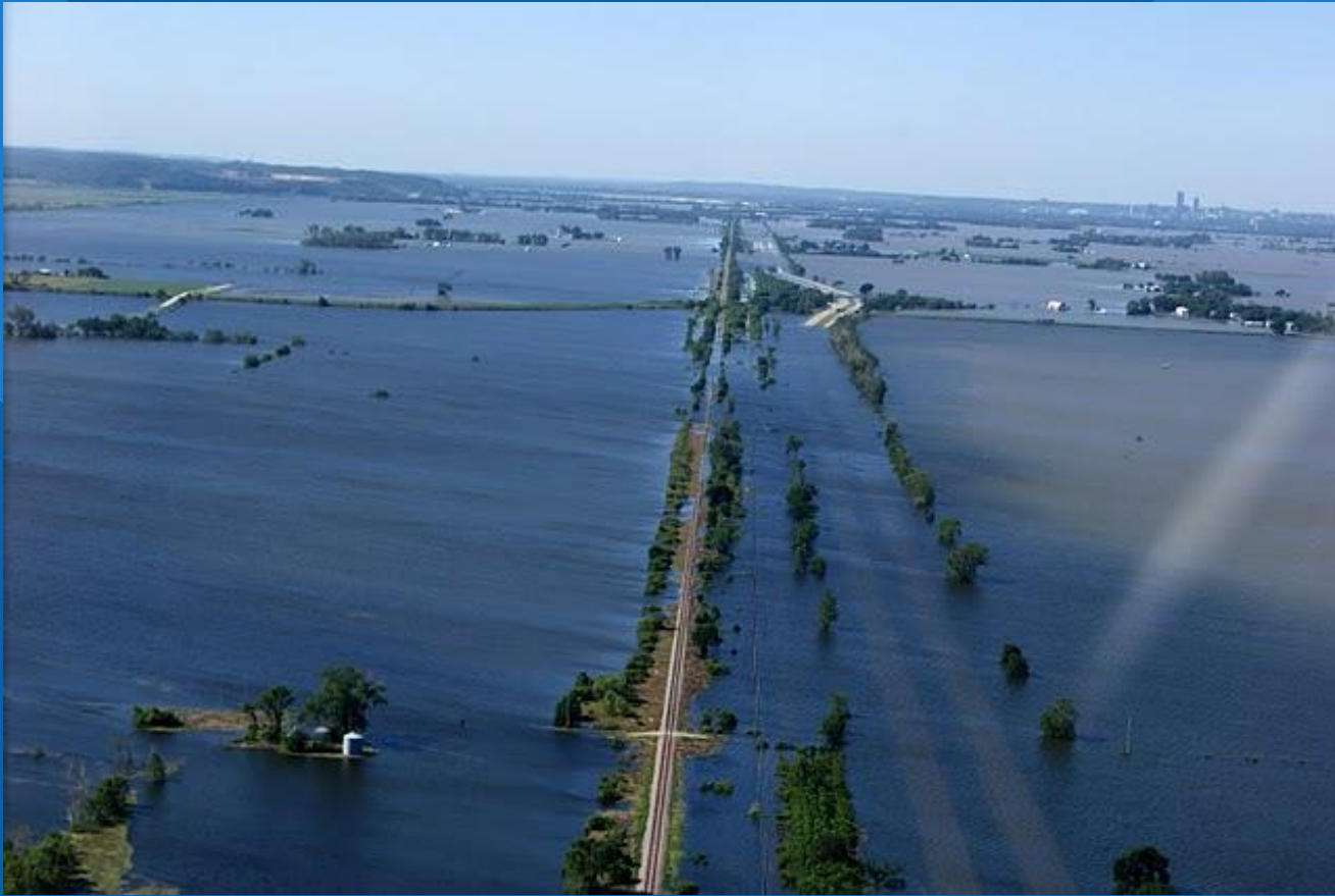
Interstate 29 underwater: Missouri River flooding in Omaha, NE June 2011. Photo by Larry Geiger. [ https://franceshunter.wordpress.com/2011/06/20/great-missouri-river-flood-of-2011/ ]
