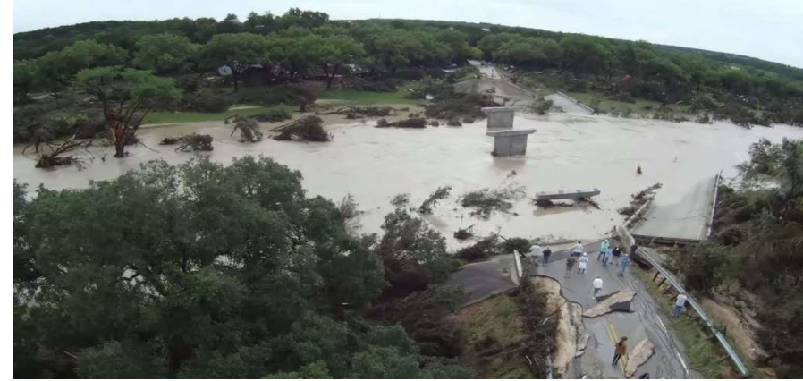
Fischer Store Bridge Memorial Day flood of 2015
