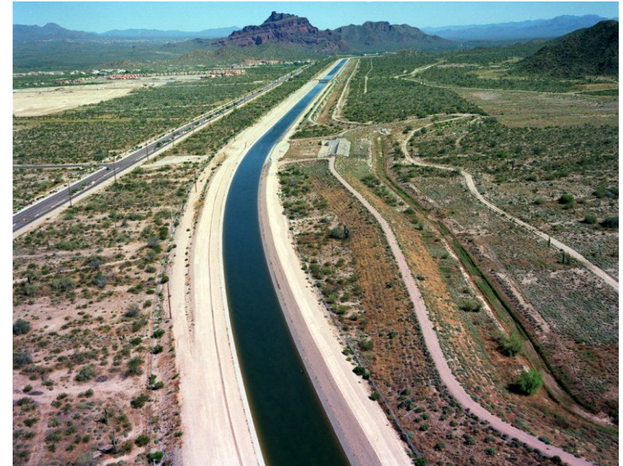
CAP Aqueduct – courtesy of USBOR
