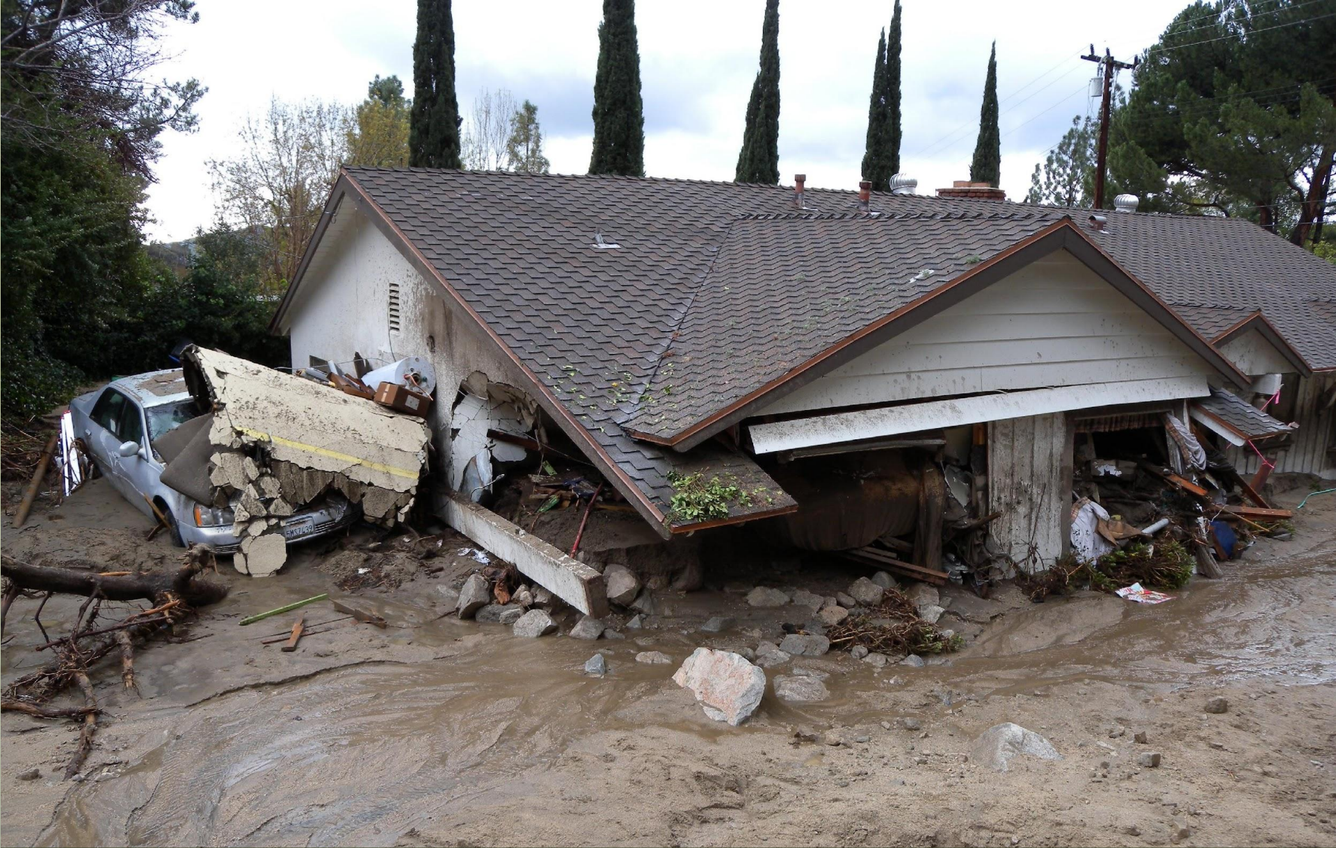
Debris Flow, 2009 Station Fire, California
